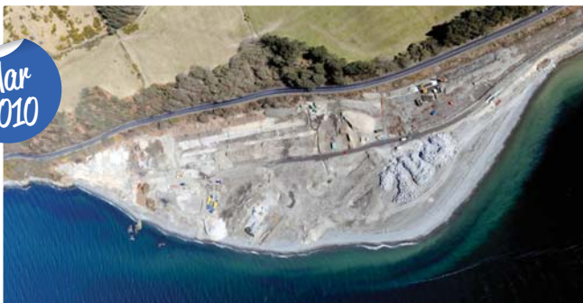
March 2010 - after enabling works have begun
